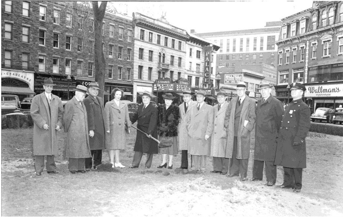
Advocate—Seaf Construction of the Stamford Service Roll started this morning with Department of Service workmen, under the supervision of Councilman Ralph Rich, member of the Service Roll Committee, making the required excavation. A concrete foundation will be constructed. The work of preparing the slats which will bear the names of Stamford men and women in service is also being pushed as is the millwork for the monument at Stamford Trade School under the direction of Frank Laney. The committee on names, Col. James Wild, Kingsley Gillespie and Samuel Morrell, is seeking the names of all Stamford people in service at any time during the current conflict. Present in Central Park yesterday as ground was broken for the Service Roll were: Left to right—Dr. Charles E. Prange, Deputy Commissioner of Finance Frank C. Langley, Commissioner of Finance Frank T. Slavin, Mrs. Bindley Gillespie, Mayor Charles E. Moore, shown wielding the spade; Mrs. David Waterbury, sr., Corporation Counsel Charles N. Wexler, Kingsley Gillespie, City Engineer Leon C. Tuttle, Lieut. Col. James H. Wild and Patrolman Asa W. Scanlon, veteran of the World War I.
