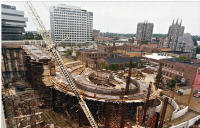
Stamford Town Center Spiral Ramp Under Construction
