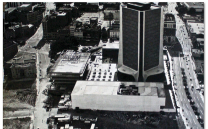
Landmark Square under Construction, The Remains of Main St. visible before being cut off
