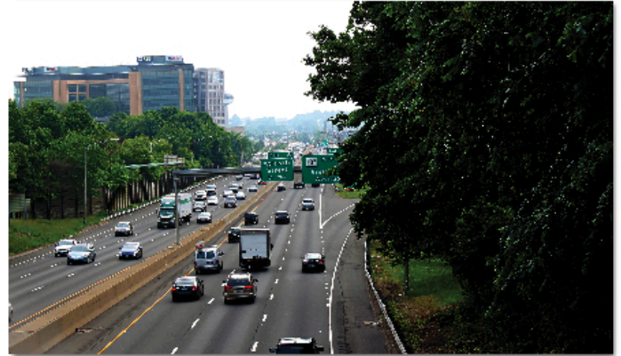
I95 North Bound Approaching Exit 7 (2016)
