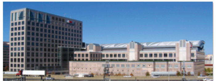
UBS Warburg North America Headquarters
