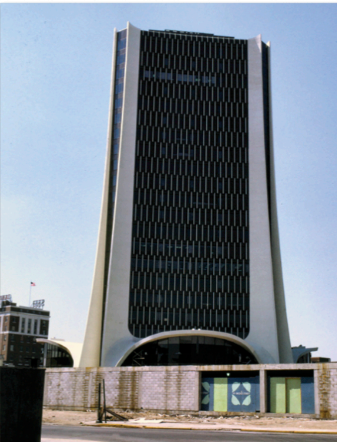
Landmark Square under Construction, View Looking North from South East
