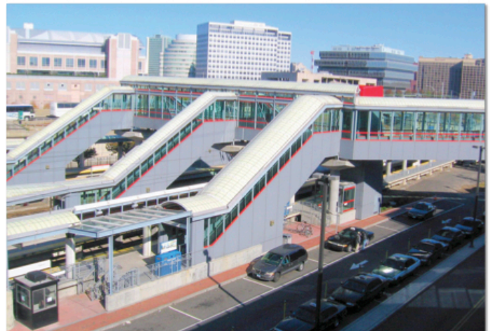
Stamford Transportation Center with Stamford's Skyline in the background
