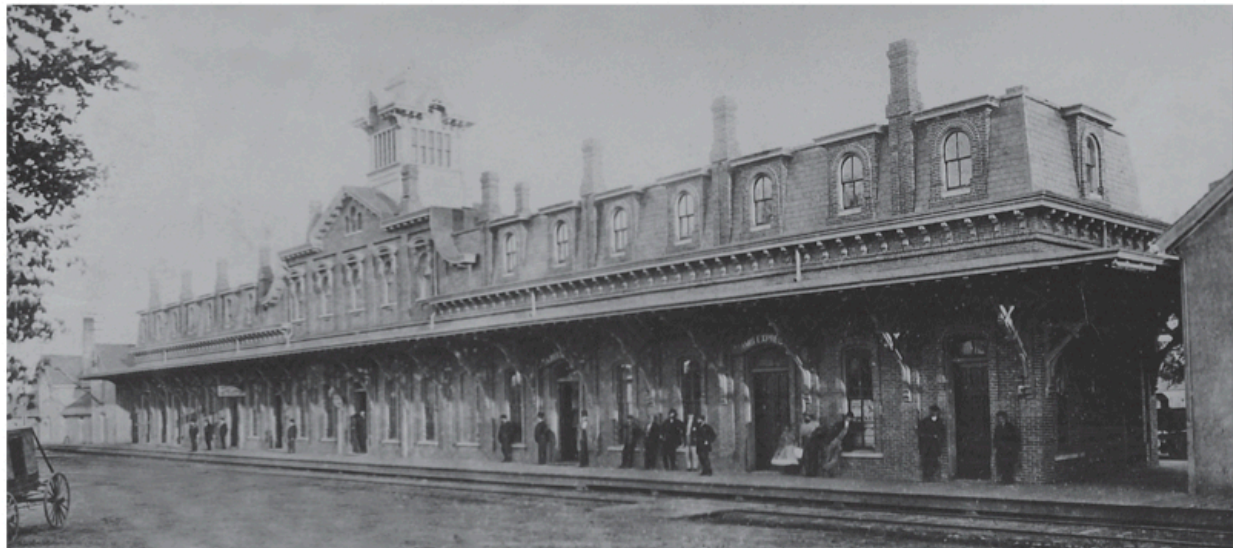
Stamford Train Station 1868
